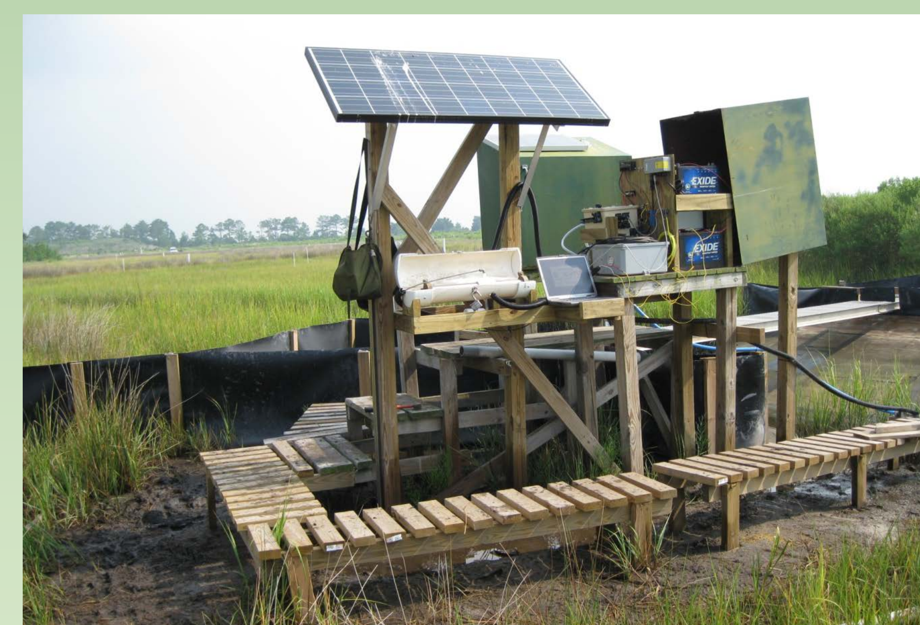
Figure 7. The downstream monitoring station in July 2011 after the spectrophotometer was removed from the stream.
